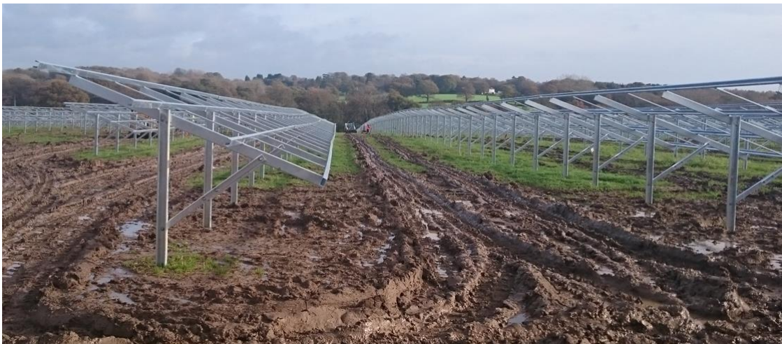
Inserts 2 and 3: Inter-row Ground Restoration
